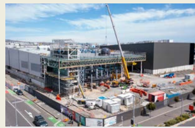
Metro Sports (Under construction)
