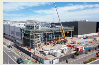
Metro Sports (Under construction)
