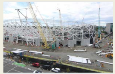
Te Kaha Stadium (Under construction)
